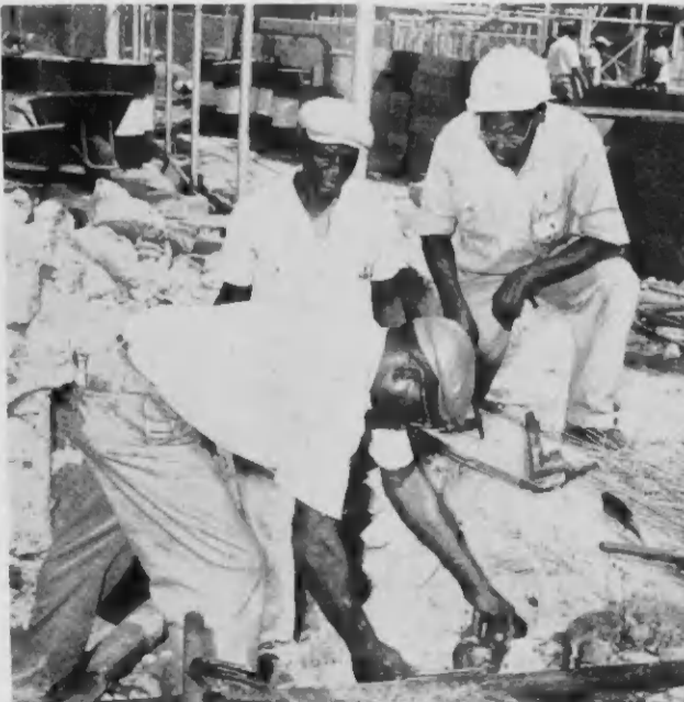
A GROUNDING system is installed by workers, above left. Others smooth poured cement before the ditch is filled, braze cables going through into the government substation grounding system, and build pull boxes through which Lago's power cables will be connected to government switching gear.
